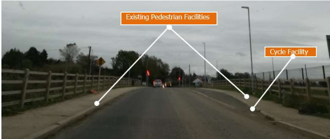
FIGURE 6-5 EXISTING PEDESTRIAN & CYCLE FACILITIES ON THE R125 ROAD CORRIDOR
