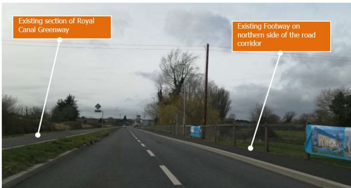
FIGURE 6-4 EXISTING PEDESTRIAN & CYCLE FACILITIES ON THE R148 MAYNOOTH ROAD
